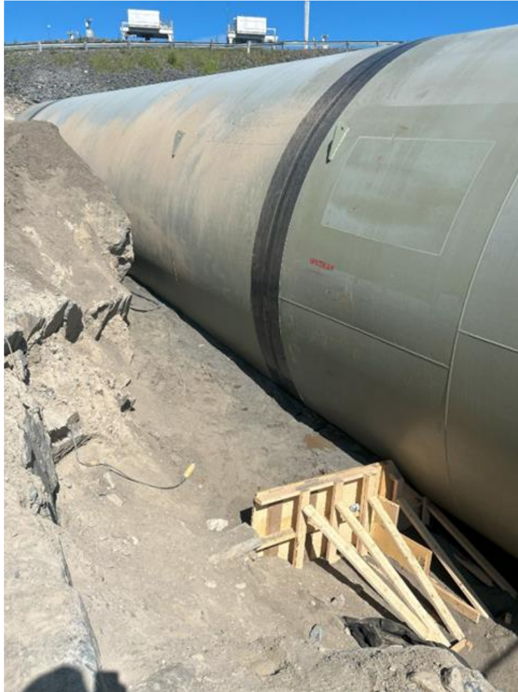
Figure 11: Exterior Coating Product on Circumferential Welds – Can 3
