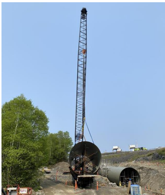
Figure 6: Preparing to Lift Can 7
